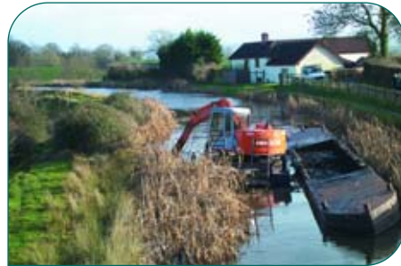
Dredging near Swing Bridge.
