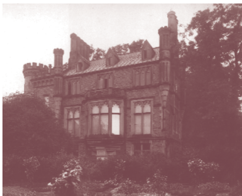
Bolton Hall before it was demolished.
