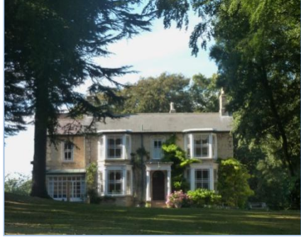
Fig. 5.2 Manor house at North Ormsby
